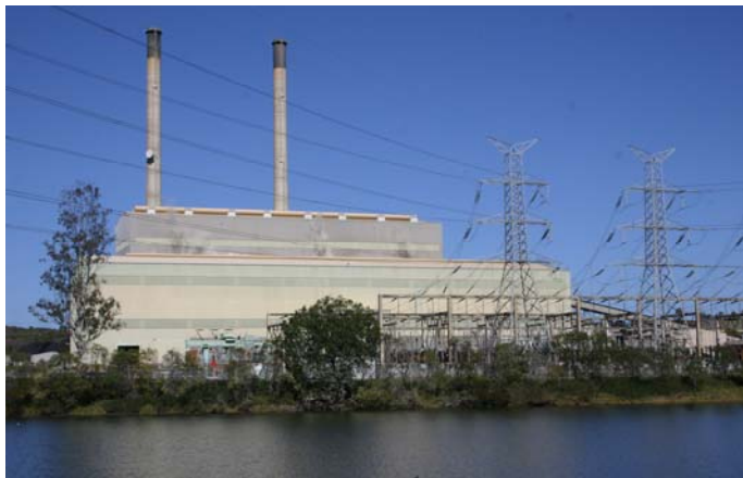
Swanbank B Power Station
