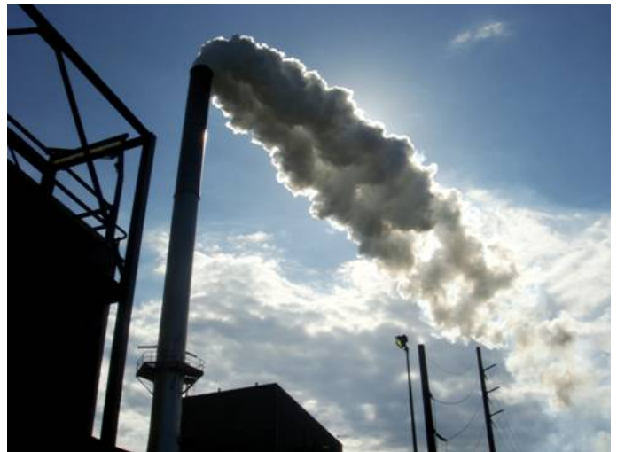
Rocky Point Cogeneration Plant
