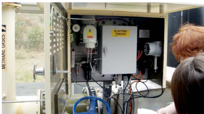
Inspecting the gas metering system
