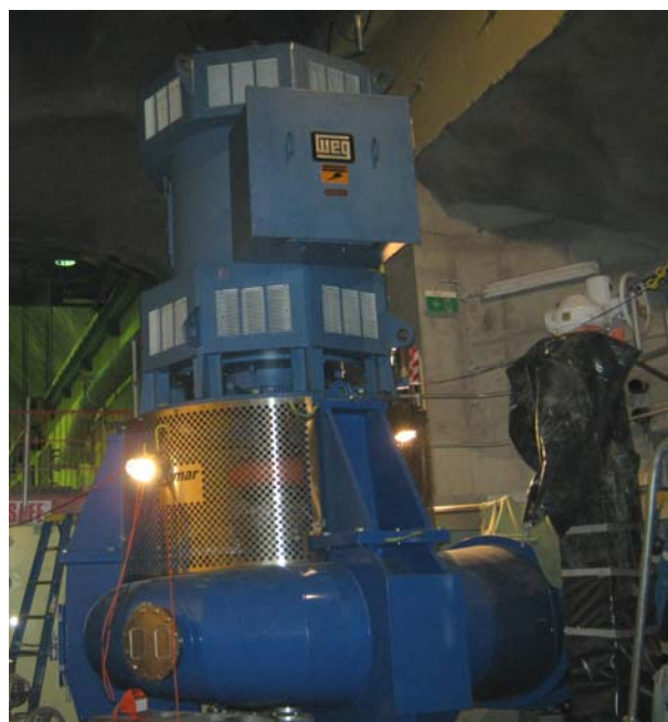
Figure 2: Hydro-electric plant being installed
